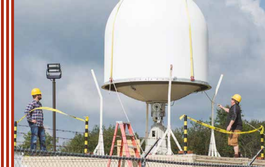
Electronics Technician Matt Mills, left, and Electronic Integrated Systems Mechanic Don Christman remove an AN/FRC-181 Milstar Air Force Command Post Terminal radome from the roof of an Extremely High Frequency Antenna Support Shelter.
