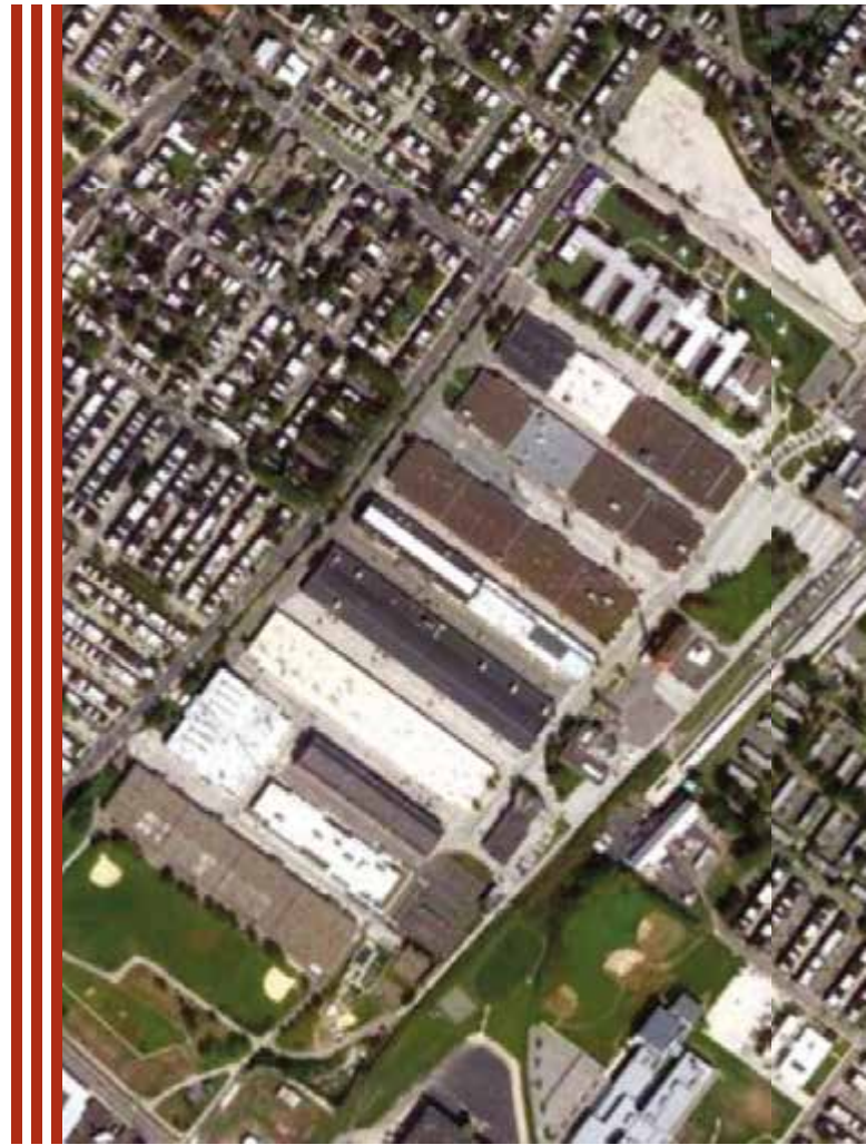
Aerial view of NSA Philadelphia's 135-acre site located in northeast Philadelphia.
